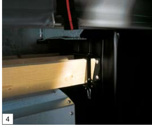
Brackets for support laths on the side of the I-beam
